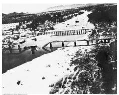
The real bridge on the "River Kwai" (actually built over the Mae Klong river). Aerial photograph shows severe damage to the middle spans caused by Allied bombing in May 1945.
